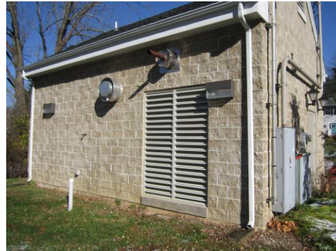
Well No. 8 Following Generator Installation
