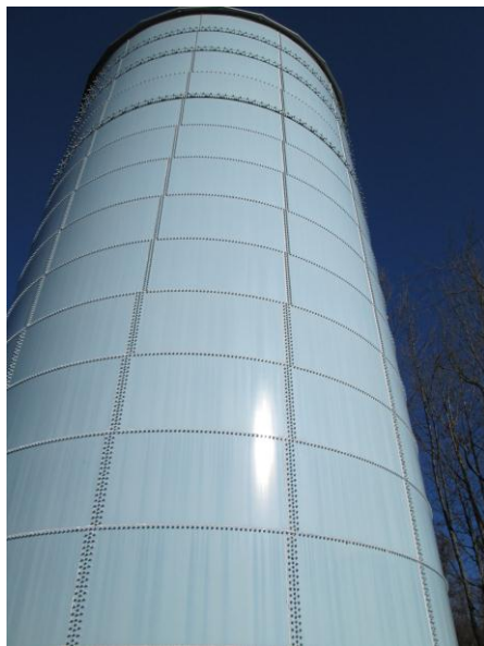
Mount Olive Township Water Storage Tank
