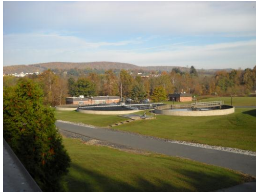
Water Pollution Control Plant Site
