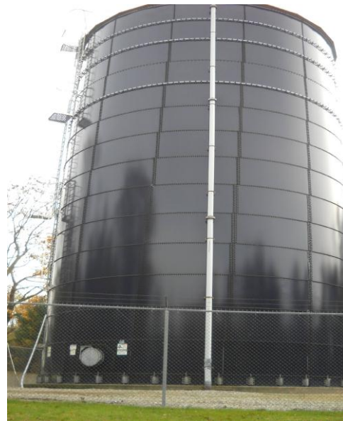
Independence Township Water Storage Tank
