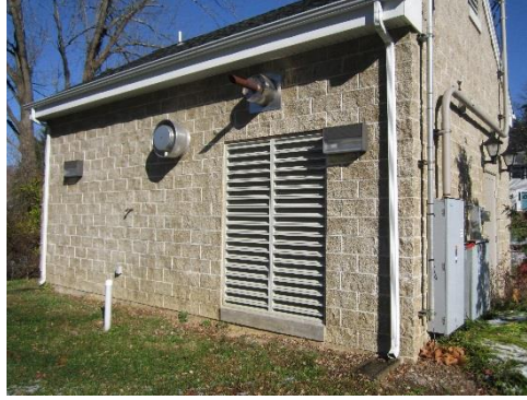
Well No. 8 Following Generator Installation
