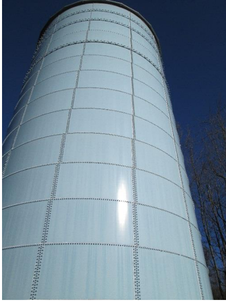
Mount Olive Township Water Storage Tank
