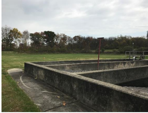
Former Equalization Basin Area (following abandonment)
