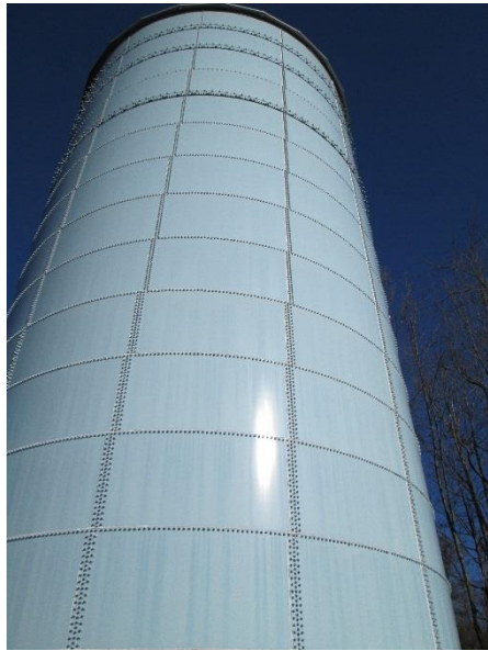
Mount Olive Township Water Storage Tank
