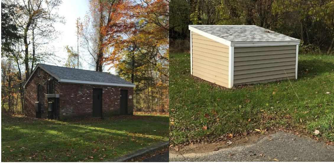
Well No. 4 New Roof Installation
