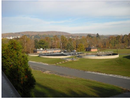
Water Pollution Control Plant Site
