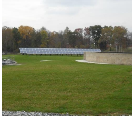
Solar Panels at WPCP Site
