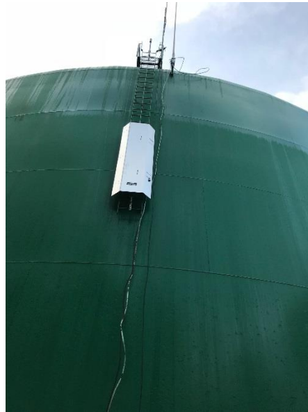
2.4 MG Tank Following 2017 Painting
