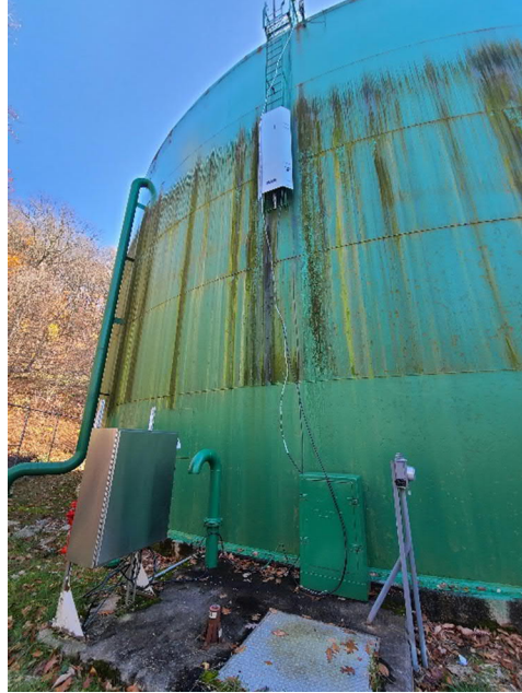
2.4 MG Water Storage Tank
