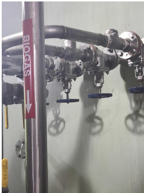
Replaced Check Valves
