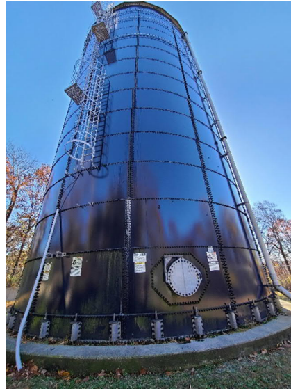
Independence Water Storage Tank
