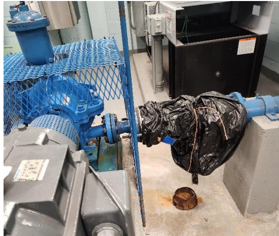
Independence Booster Station – Pump #2 Flexible Coupling
