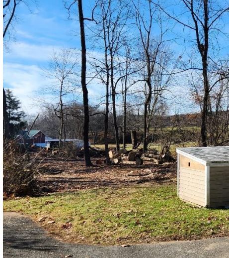
Tree removal at Site
