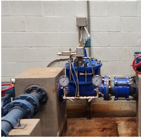
Independence Booster Station – Altitude Valve
