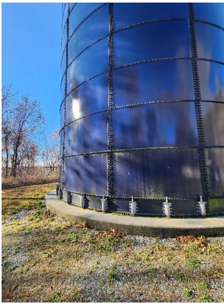
Independence Water Storage Tank
