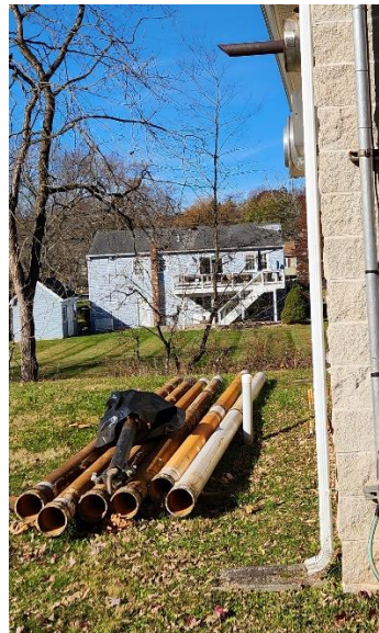
Pipes behind building
